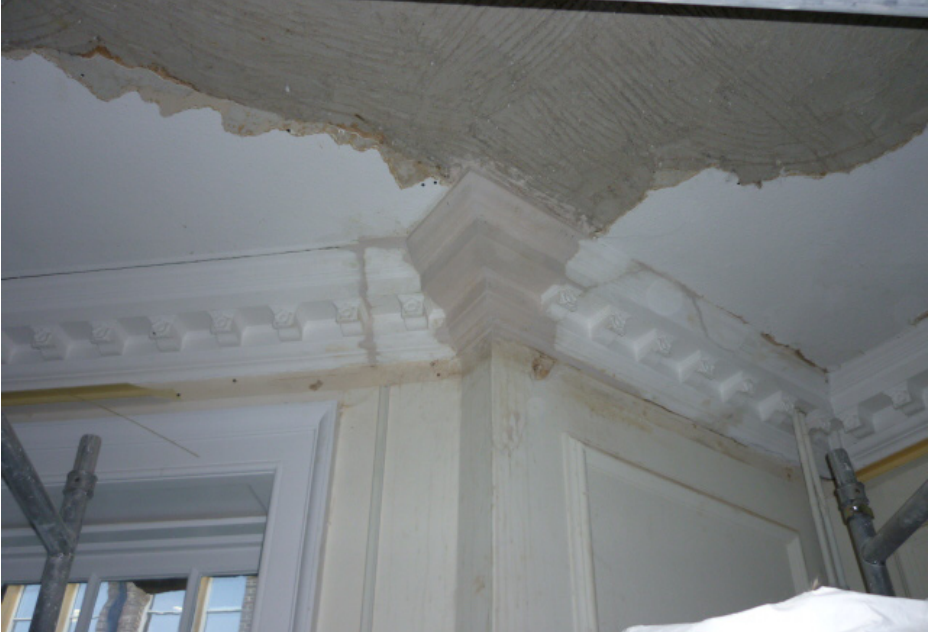
Lime plaster to ceiling and cornice detail
